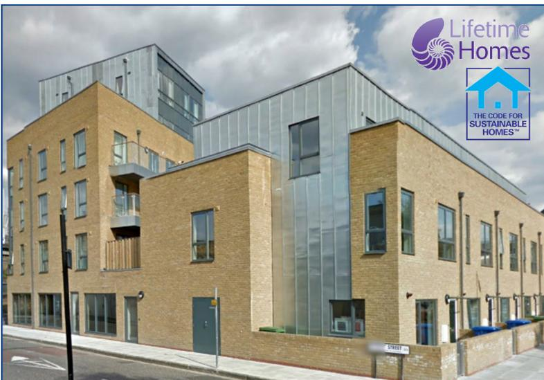
From the outset issues of constrained space and noise pollution were of paramount significance. As a Willmott Dixon Category A Supply Chain member, Russell Timber Technology's Timber Alu-Clad Premium Performance Doors and Windows were used to address the issue of rail traffic sound with a minimum Acoustic protection of 44db and U-Values of 1.2.
